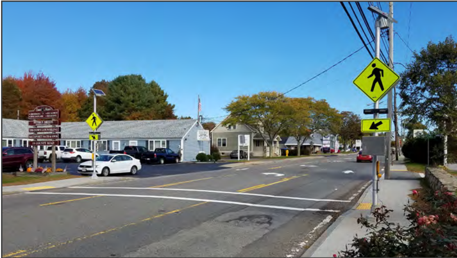
Rapid Rectangular Flashing Beacons (RRFBs)
