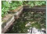
Bell Rock Rd crossing Queen Gutter Brook. Near Wilson Rd. Shows Public Supply Water.
