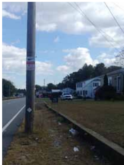
Photo 4: Bus stop without a connection to sidewalk network
