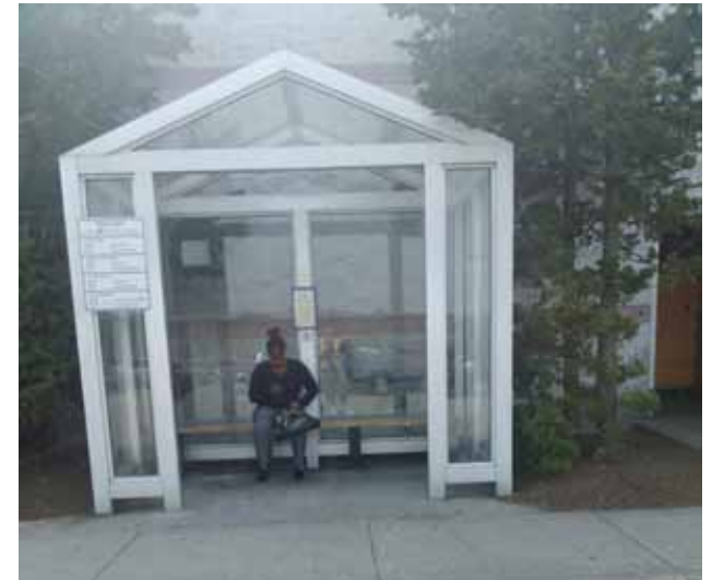
Photo 9: Bus stop with shelter and route information sign
